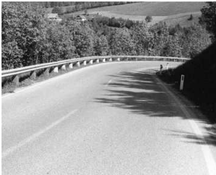
An Austrian road with a crash barrier fitted with CBP polystyrene impact attenuator
